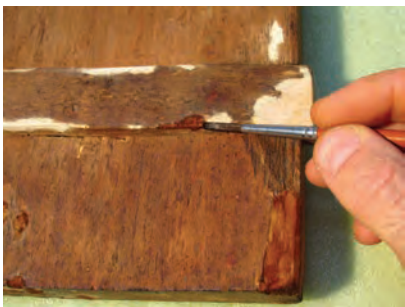
▲ Fig. 20. Chromatic integration of new pieces of wood.
