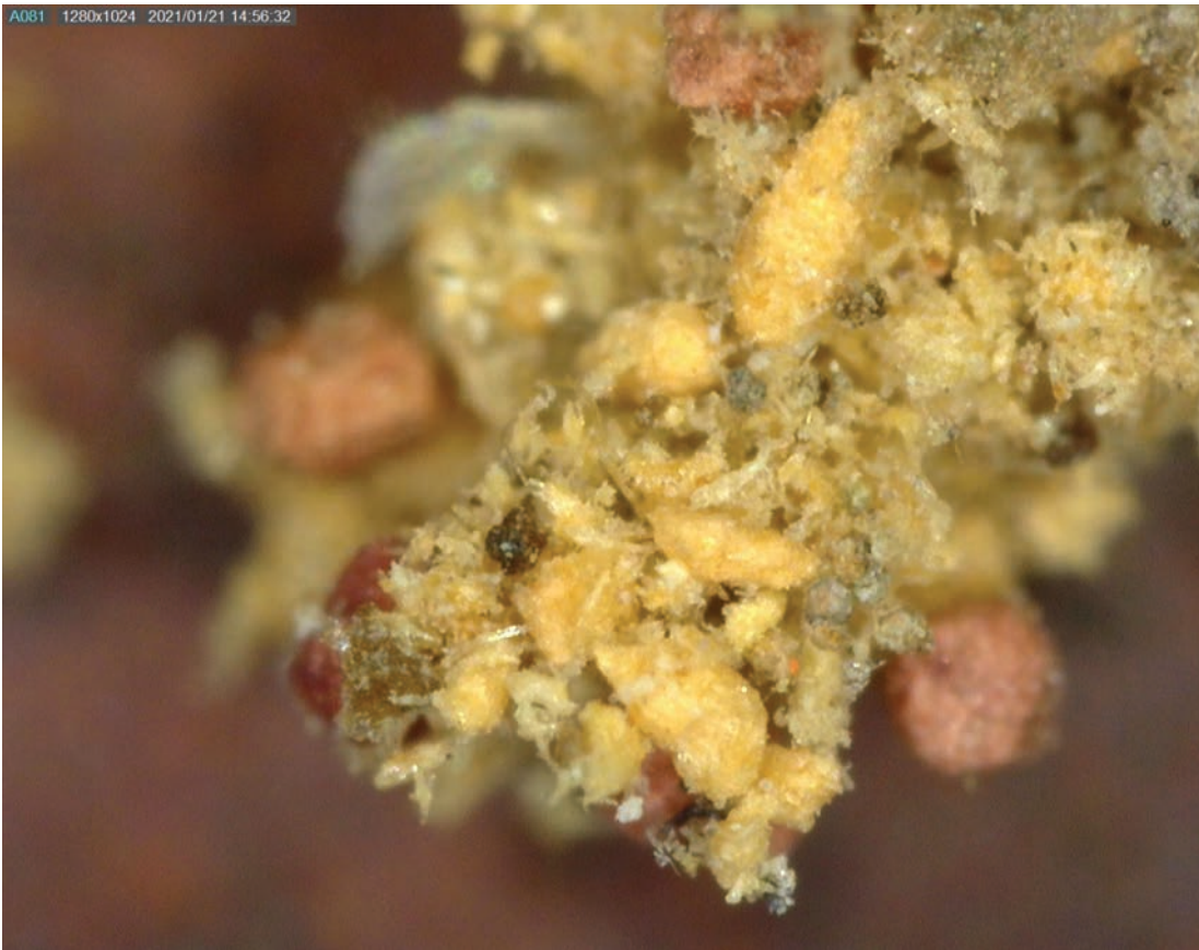
◆ Fig. 12. Details with the tunnels made by insect larvae in the wooden structure and fly holes that weakened the structural stability of the wooden panels, and microscopic details of the fly holes. Credits: Dumitrița-Daniela Filip.
