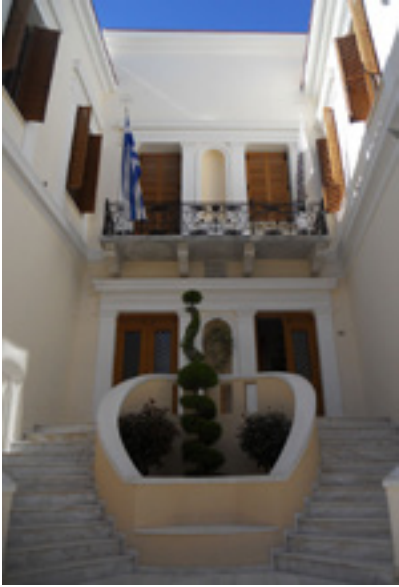
Fig. 5. Episcopal mansion of Rethymno, funded by the Russian administration of the city in 1900. Photo S. Katopi
