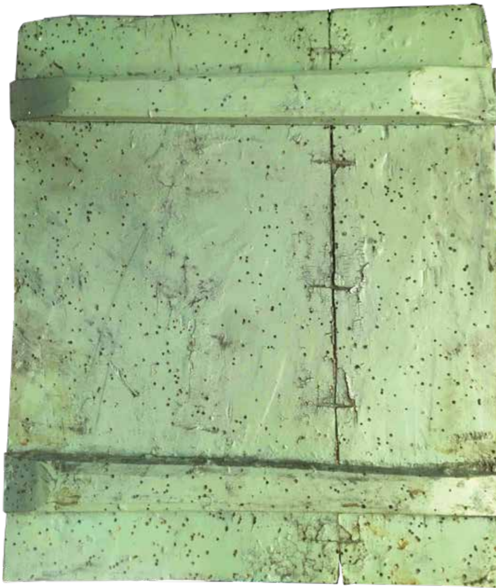
Fig. 19: Metal staple reinforcement. Photo: A. Nikolov.
